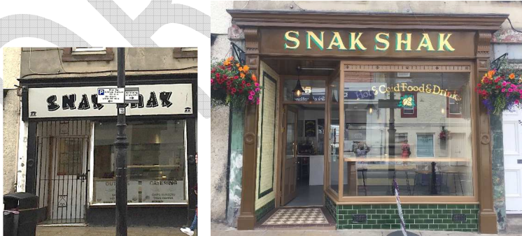
55 High St: Before improvement
