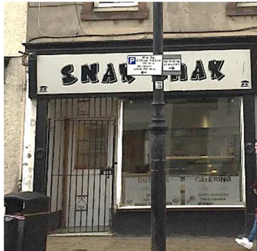
55 High St: Before improvement
