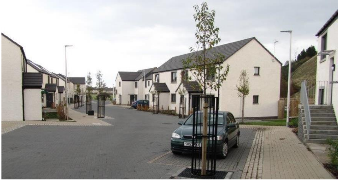
Affordable housing in North Berwick
