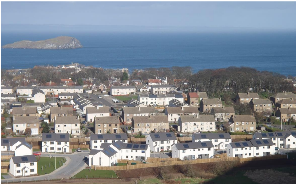
New Council Housing at Law View, North Berwick
