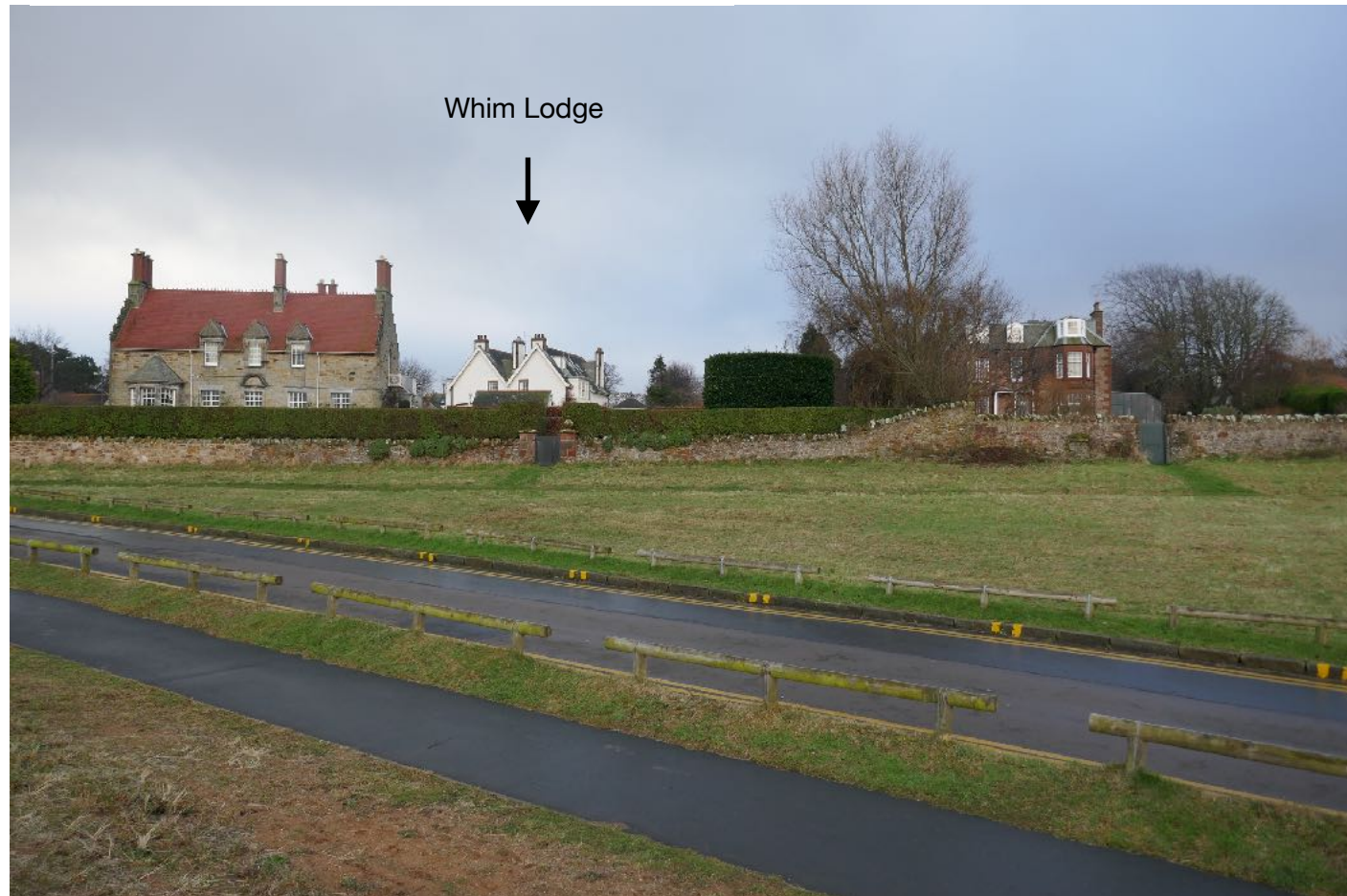
FROM BY THE CAR-PARK ACCESS ROAD
