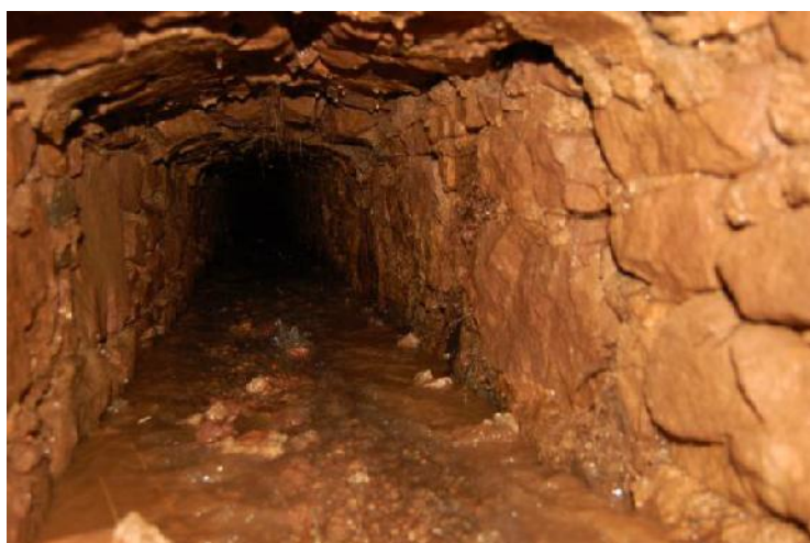
Figure 4 - Culvert interior
