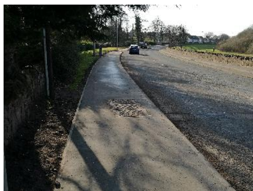
A iii – looking southwest down A1087
