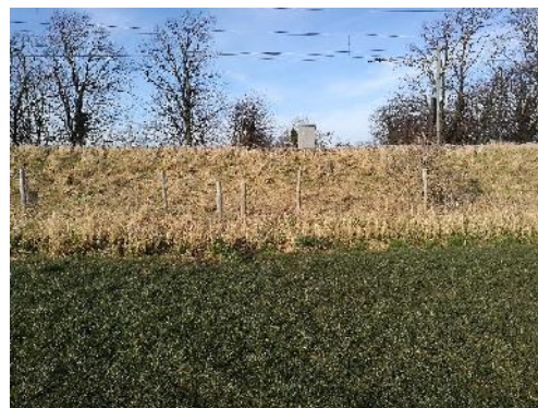
B v – Looking southeast over railway line
