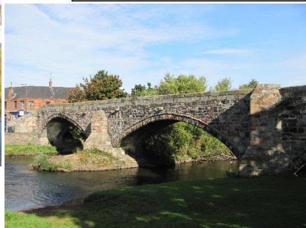
Roman bridge linking built form of the town into the natural river area
