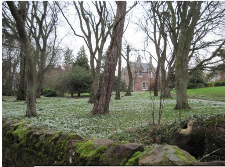
B-listed Pitcox Farmhouse set in wooded grounds surrounded by moss covered boundary walls typical of the area
