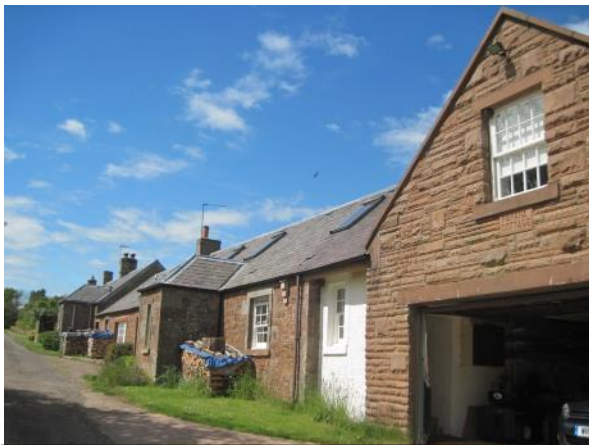
Traditional stone and slate cottages at Snawdon, sensitively extended
