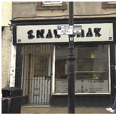
55 High St: Before improvement
