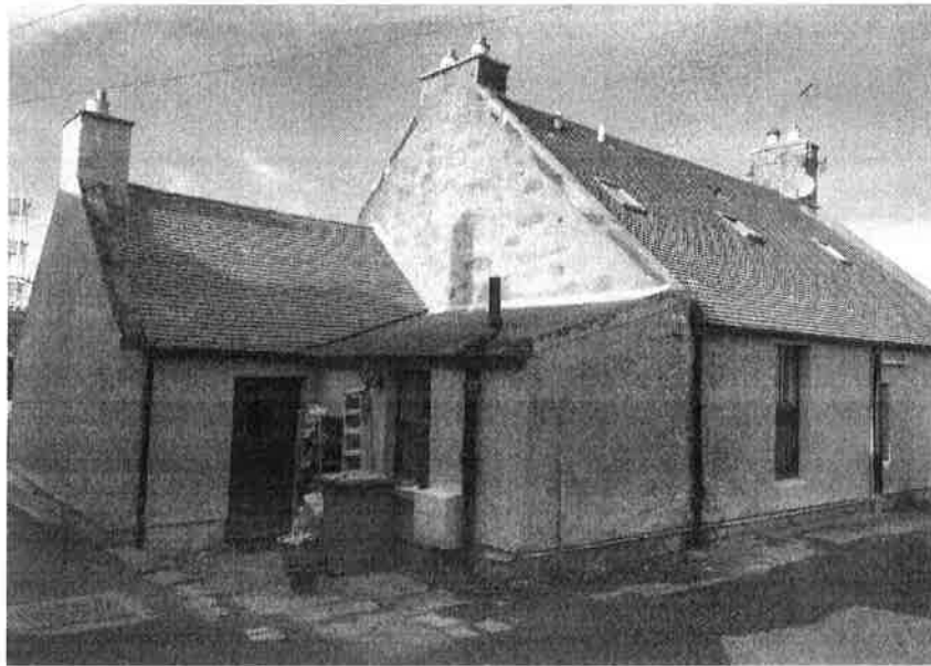
Rear View – The kitchen annex has a proposed rooflight and roof vents to match the existing. The small WC window on the far right will be replaced with a timber double glazed unit to match the existing.
