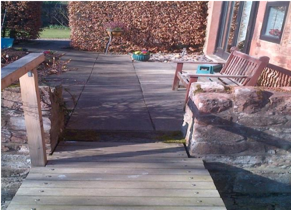
Lade Gate opening – requires Flood Barrier
