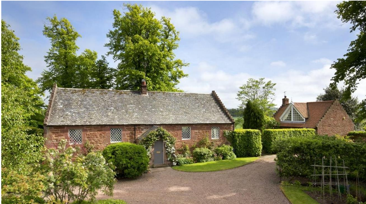
Mill and Cottage Buildings Presently
