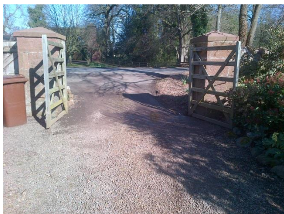
Entrance Gate requiring flood protection consider removable barrier -
