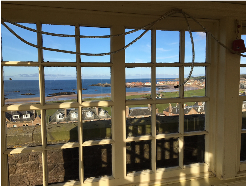
Photograph 6: View obscured by lattice of existing astragals
