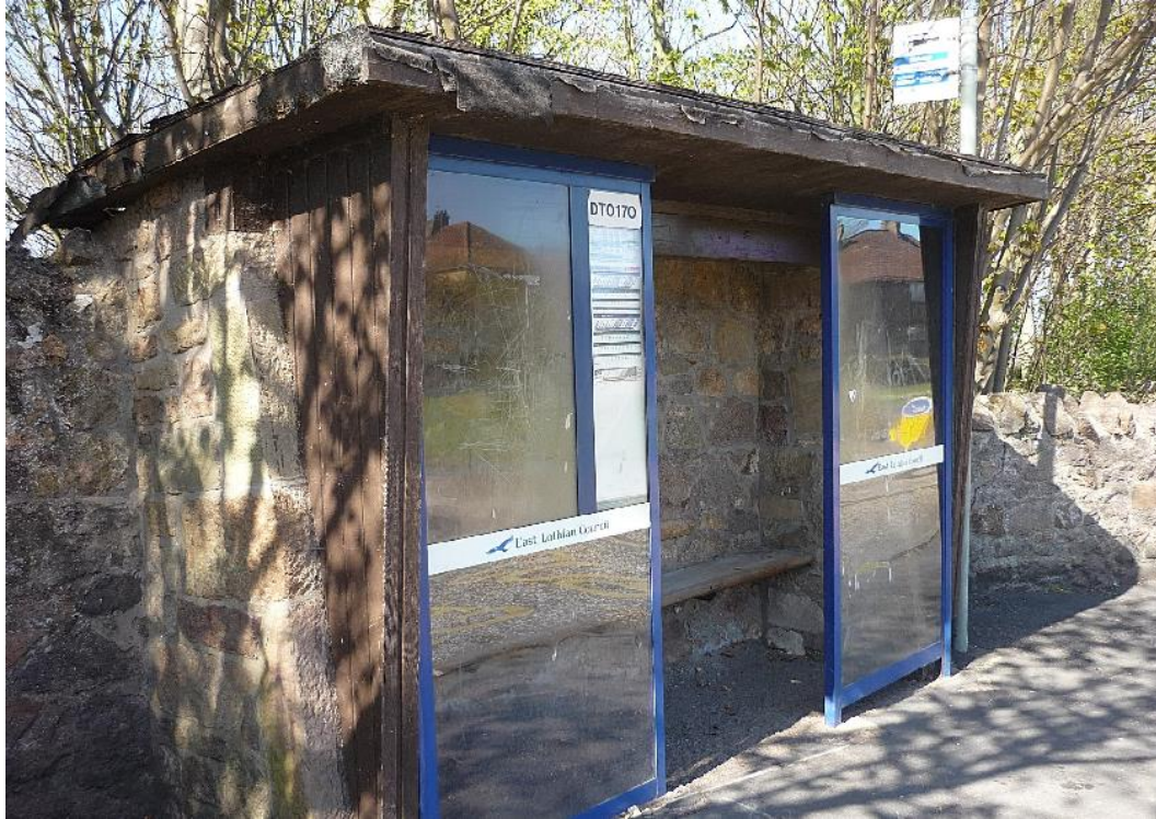
Repairs to Bus Shelter
