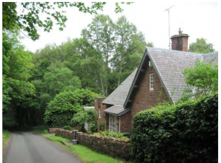
One and a half storey sandstone cottage fitted into the landscape
