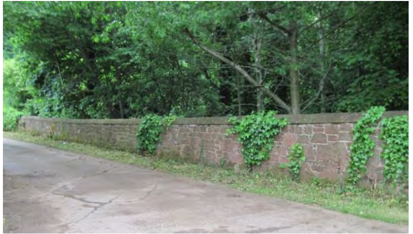
Typical red sandstone wall to bridge
