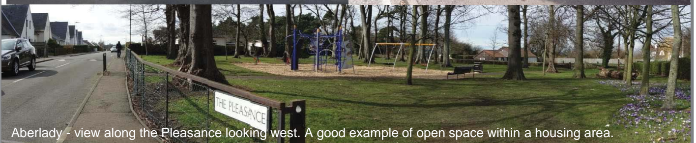
The Pleasance also has attractive 1.5 storey houses with sweeping slate roofs and vertical emphasis windows. Hedges form attractive boundary features
