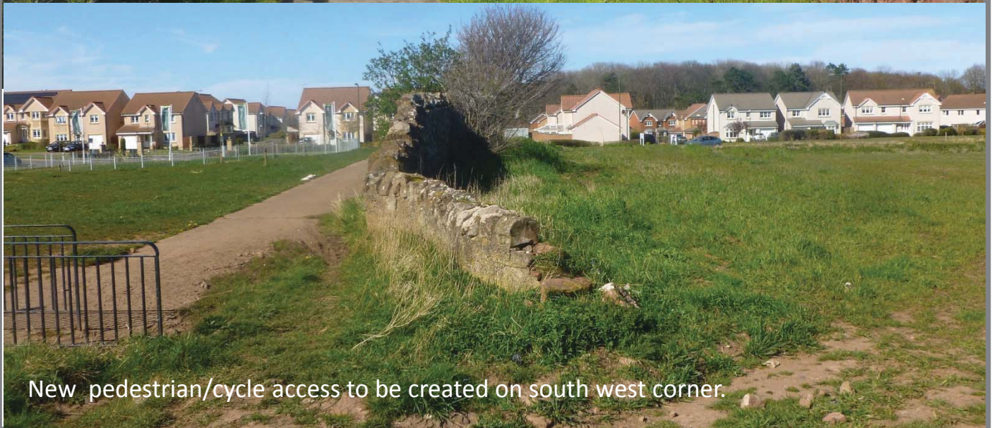
Stone wall on southern boundary.
