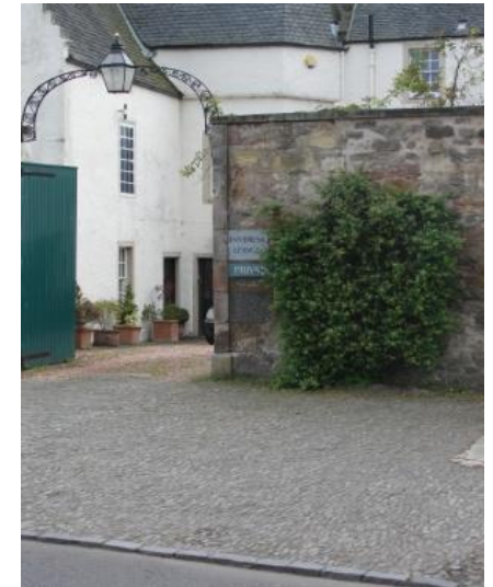
Figure 95 Good quality traditional hononised paving is important to the area and should be retained where it exists
