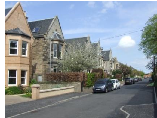
Figure 97 New houses designed to fit sympathetically with older Victorian designs on Smeaton Grove
