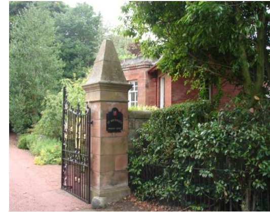
Figure 86 Stone gatepier at St Michael's House
