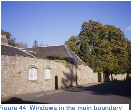
Figure 44 Windows in the main boundary walls indicate buildings behind
