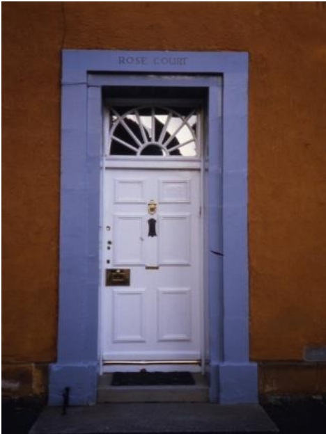
Figure 93 A grand Georgian doorway with decorative fanlight
