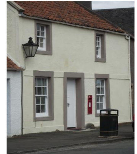
Figure 99 The former shop, after being sympathetically restored with the original window styles and with a revised colour scheme, has enhanced this part of Inveresk
