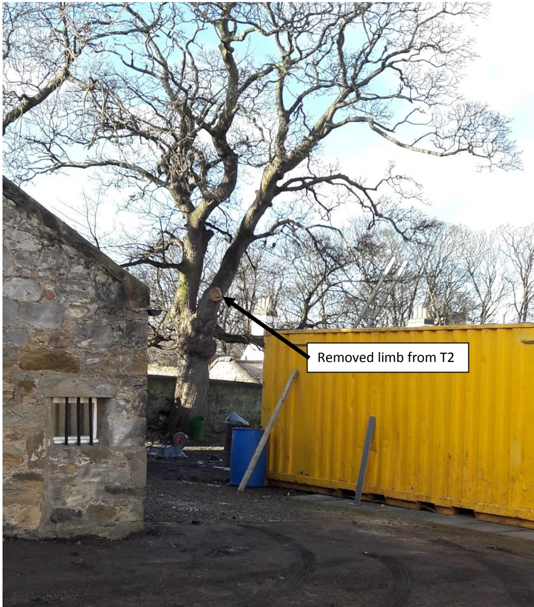
Fresh tree work to remove limb off tree T2 sycamore without notification.
