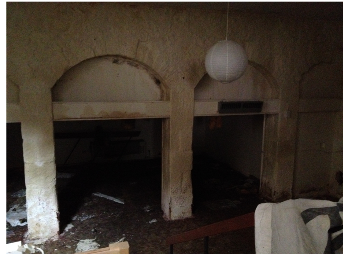
Coach House Arches - Condition Survey Photo
