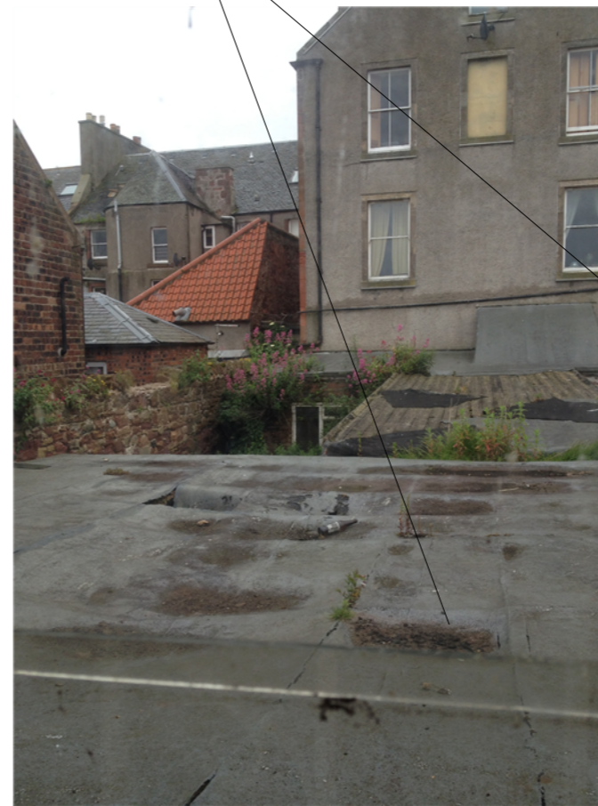
Condition Survey Photo
