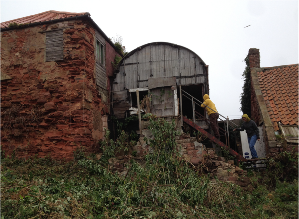
South East - Condition Survey Photo
