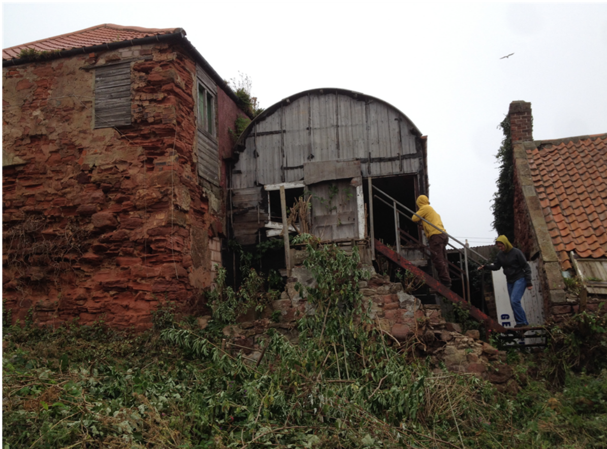
South East - Condition Survey Photo
