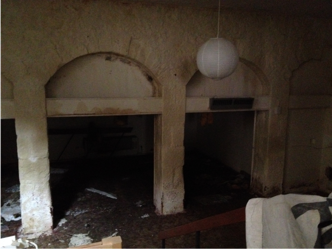
Coach House Arches - Condition Survey Photo
