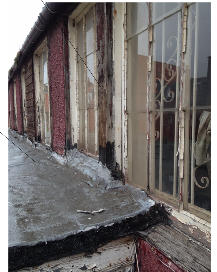
Condition Survey Photo
