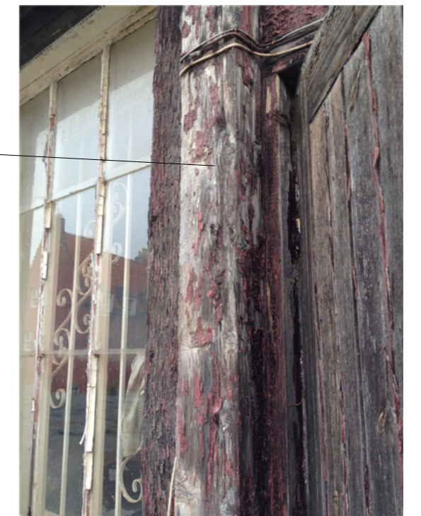
Condition Survey Photo
