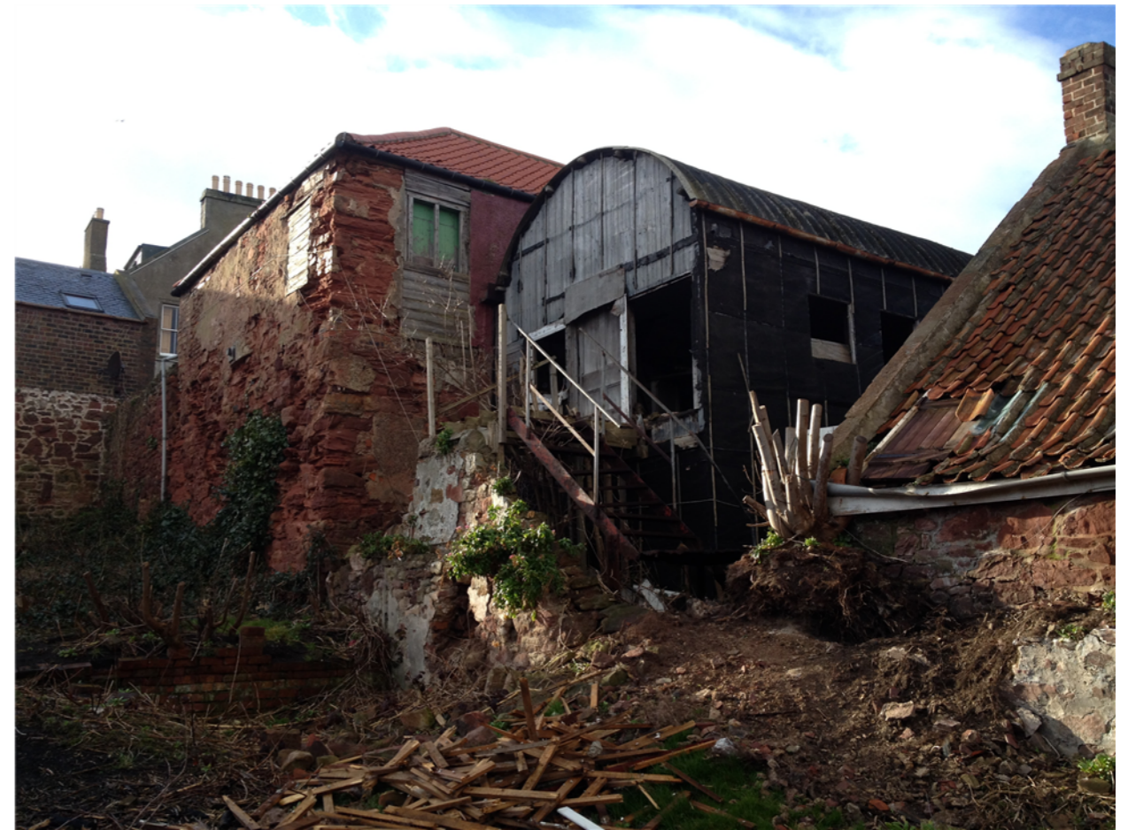
Condition Survey Photo
