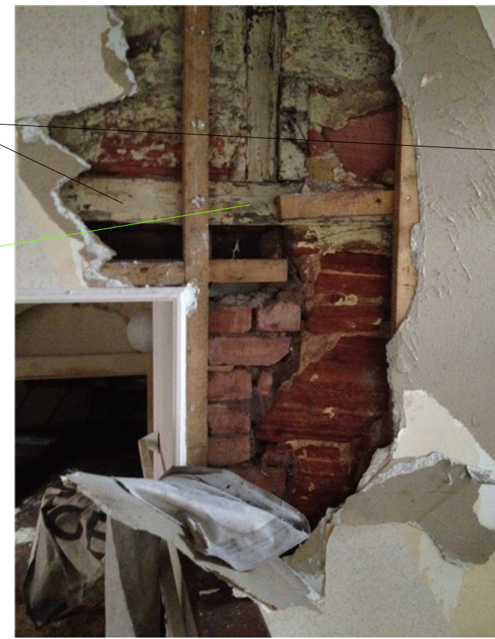
Condition Survey Photo
