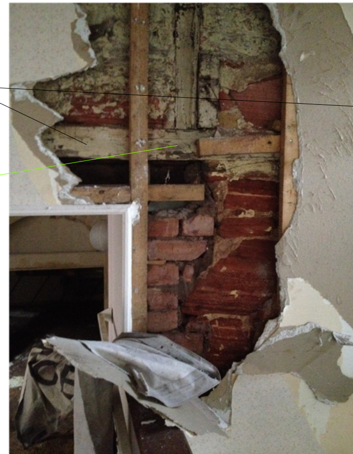
Condition Survey Photo
