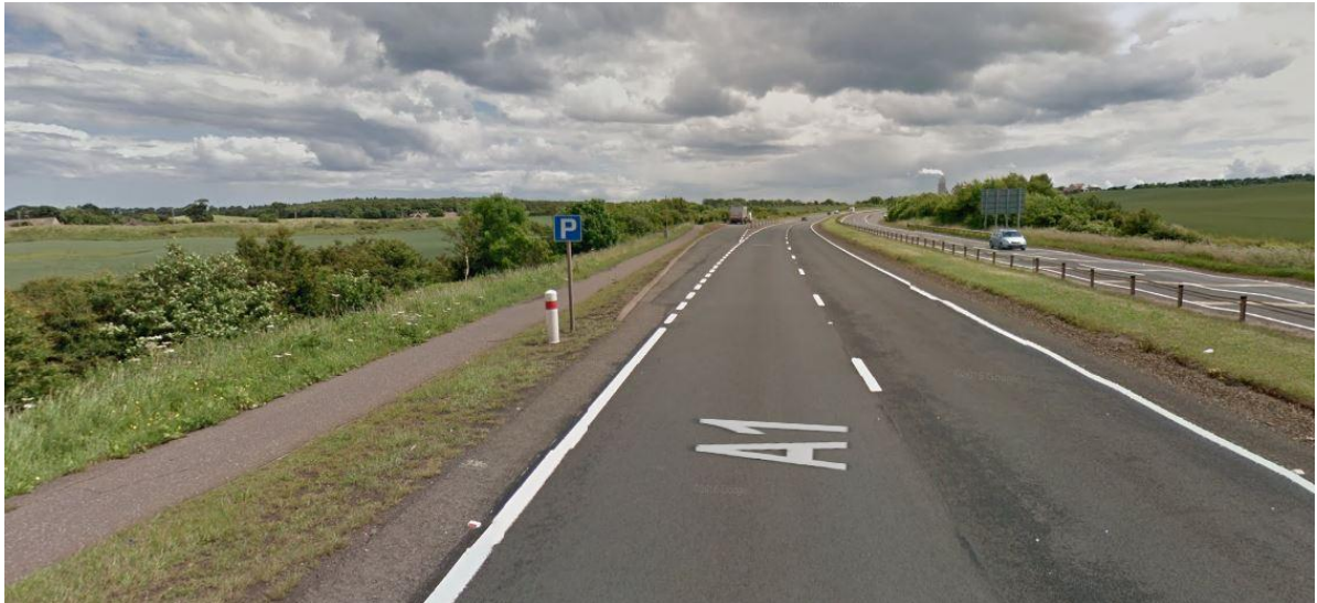
Figure 6 - Existing Parking on the A1
