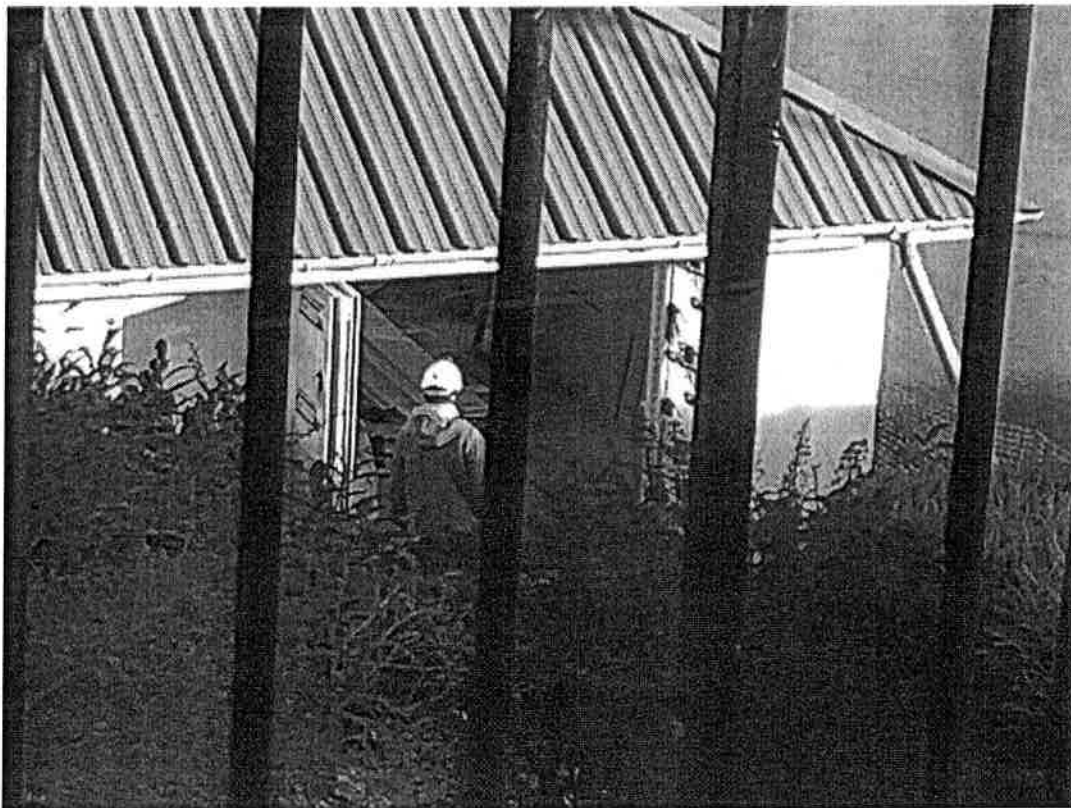
Photograph 2 :- View from Macnair Avenue lounge showing the patio door in the south wall of the clubhouse.
