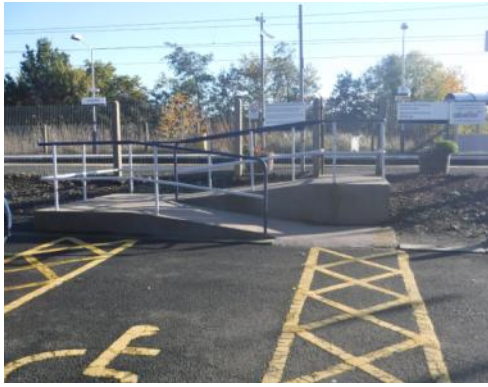
Fig. 8 – Disabled Access to Platform
