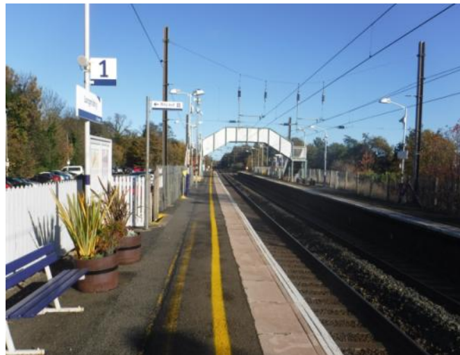
Fig. 7 – Platform 1 & Footbridge to Platform 2
