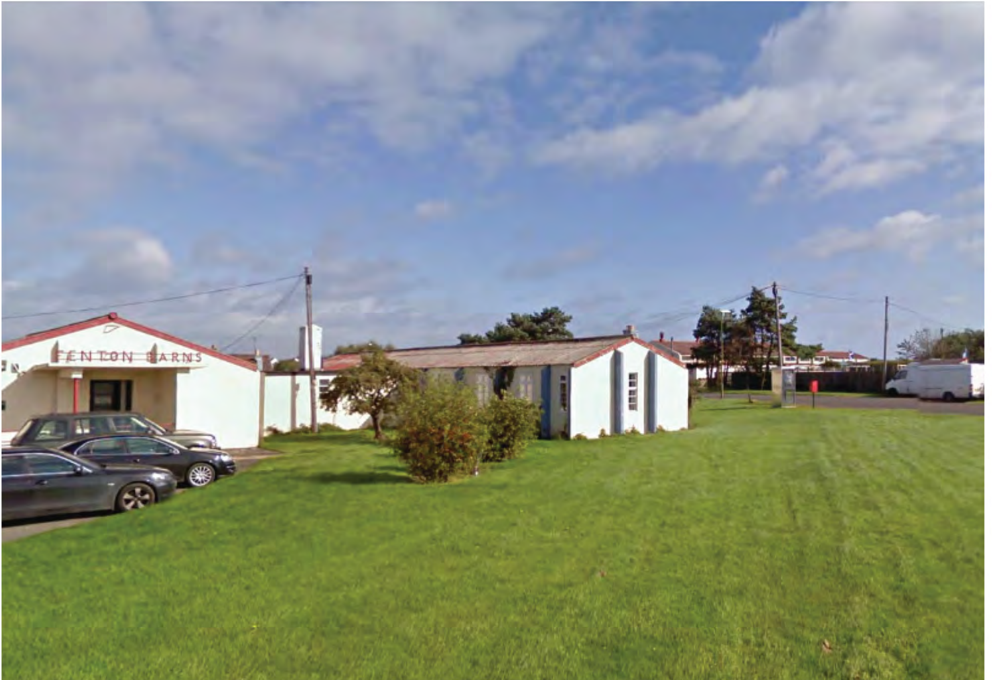
Existing buildings will form the core of a expanded village at Fenton Barnes
