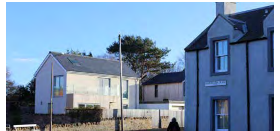
Recent housing at the foot of Haddington Road / Haddington Place
