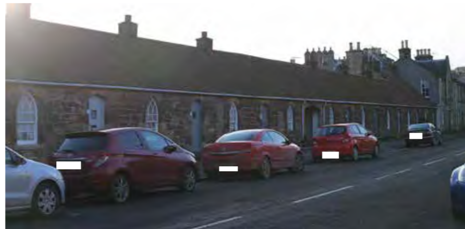
18th Century terraced cottages
