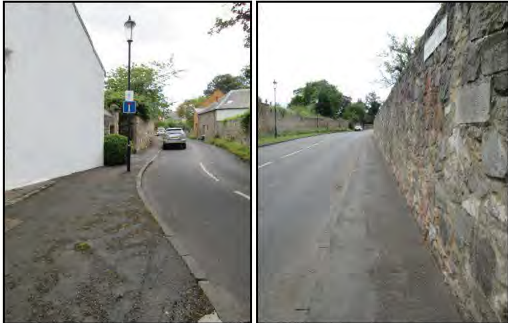
Existing footway provision at the A6124 Carberry Road / Crookston Road junction ( left ) and on Carberry Road ( Right )
