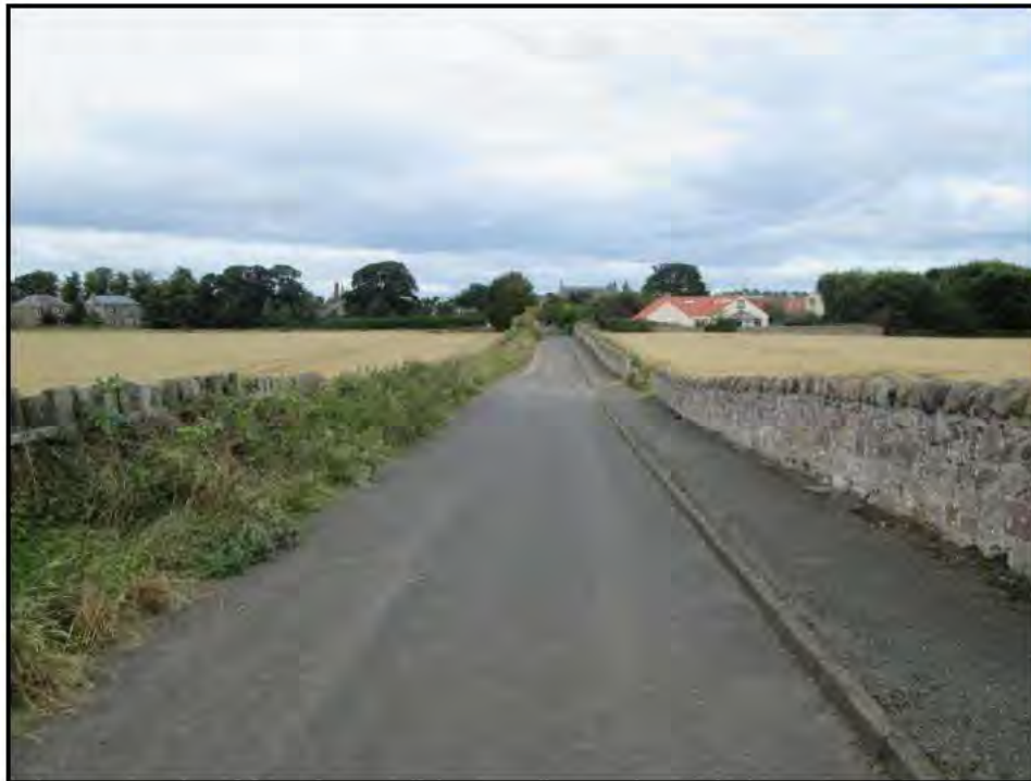
Crookston Road at the development frontage looking north
