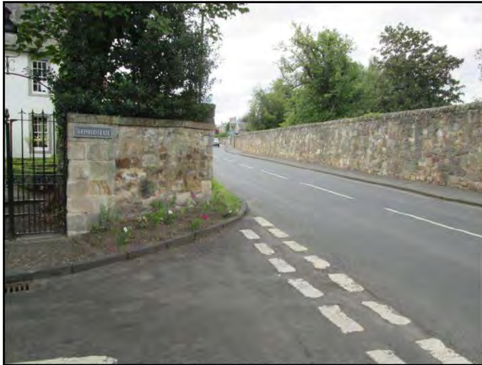
Visibility along the A6124 Carberry Road from Crookston Road
