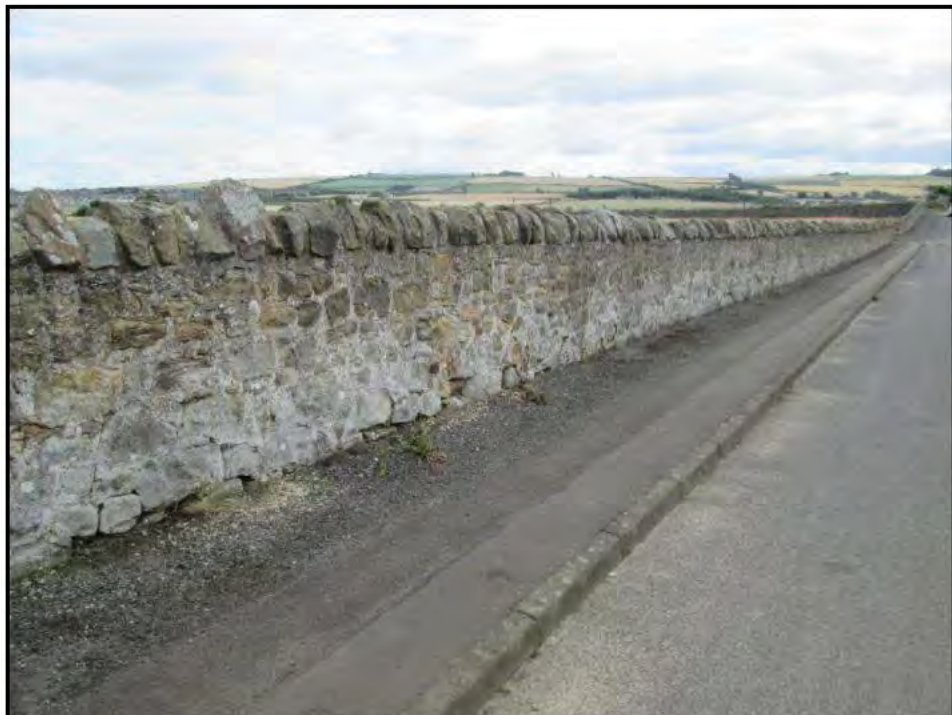
Existing footway provision on Crookston Road at development site
