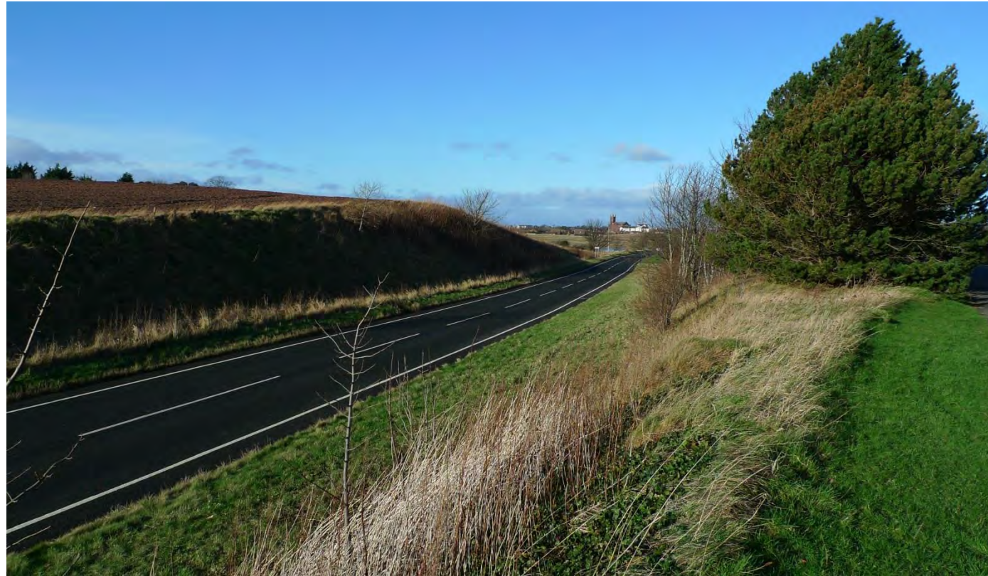
A1087 with high ridgeline of site above roadside embankment. Focal skyline feature of church prominent in view northwards.
