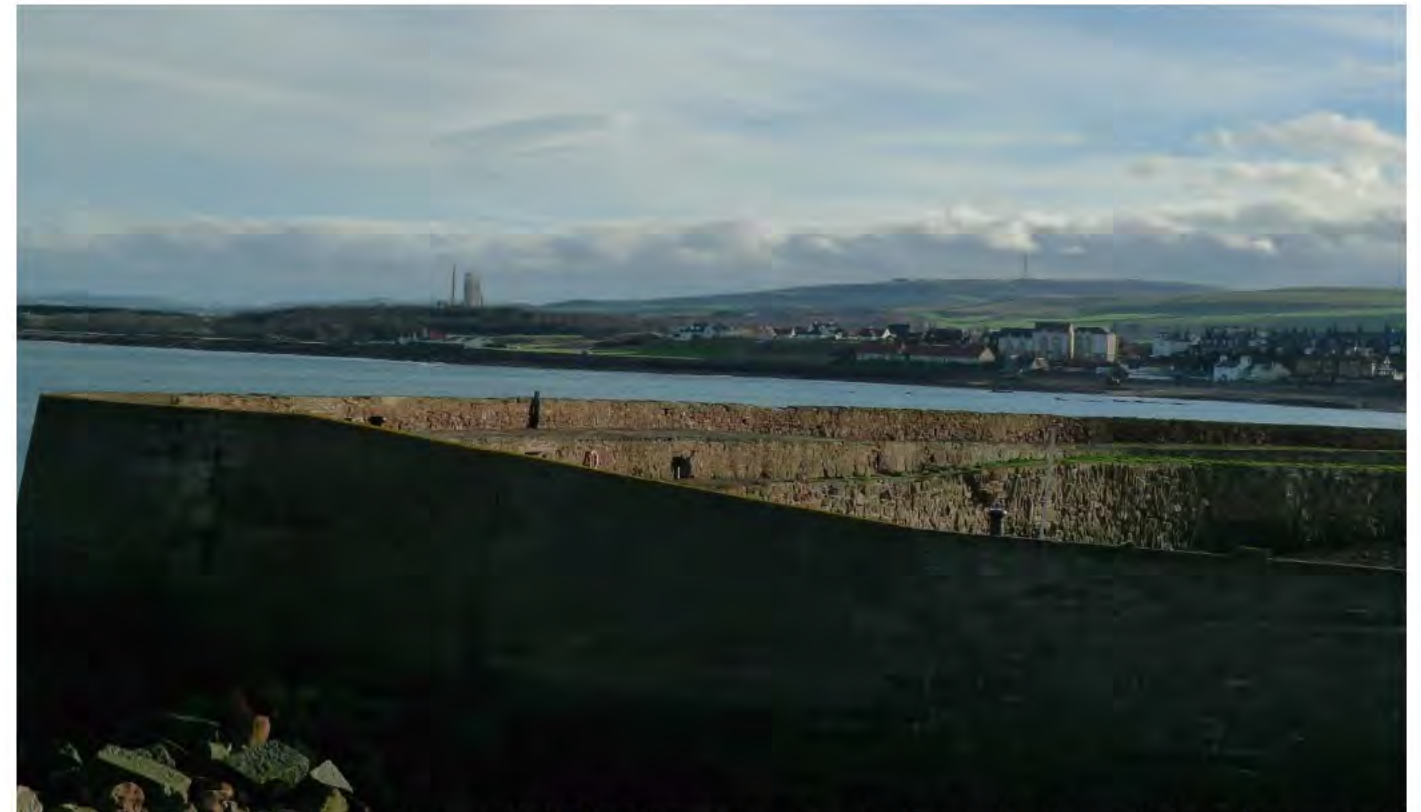
View from Dunbar Harbour. Broxmouth GDL policies form a key landscape feature, with the site screened from view by intervening buildings and woodland.
