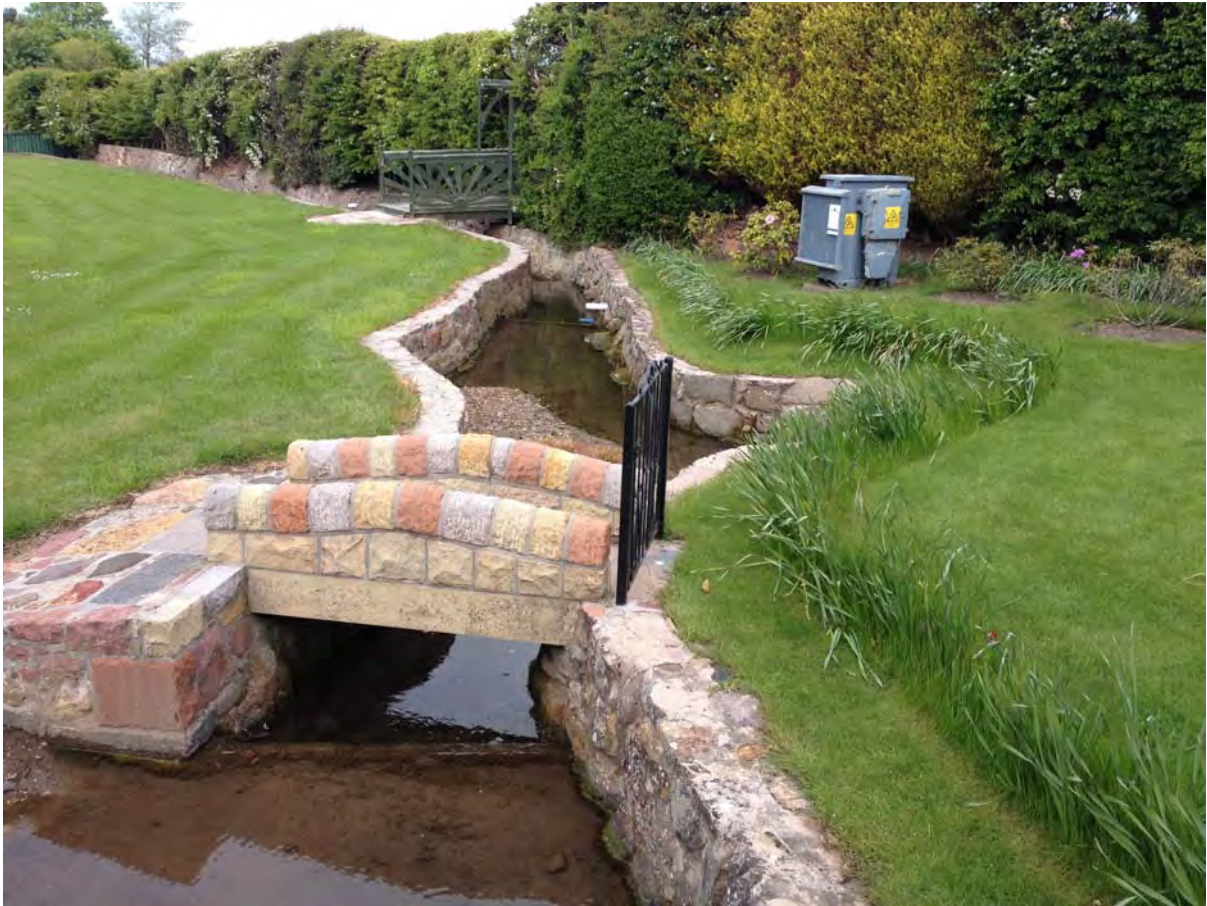
Photo 3: Watercourse flowing northwards from culvert outlet
