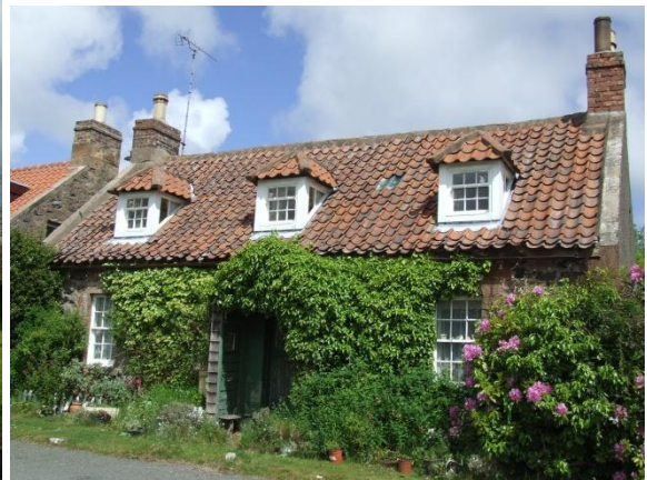
Main street through Oldhamstocks with vernacular cottages with sandstone walls and pantile roofs
