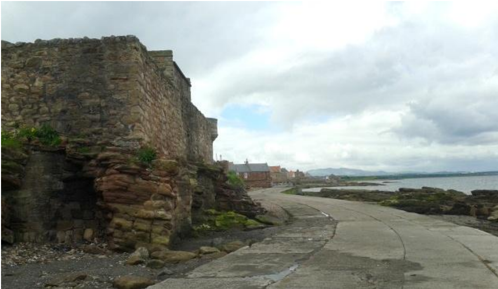
Open views along the coast to the hills of the Pentlands and Arthur's Seat in the distance and Rock Cottage sticking out in the middle distance
