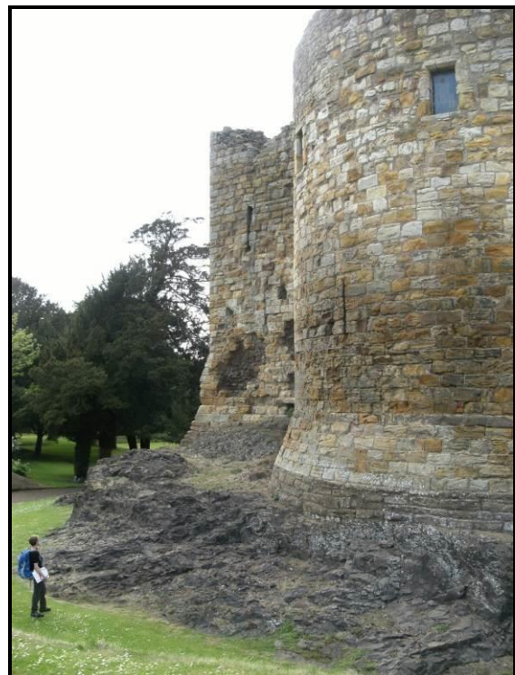
Photo ELC_10 P4: The trachyte is more blocky in appearance to the south and west of the site. © BGS, NERC.
