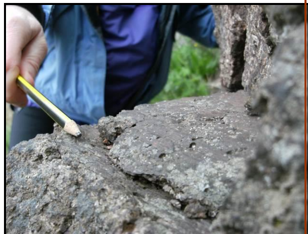
Photo ELC_7 P5: Slickenlines on joint within basalt. Slickenlines are 'scrapes' left on joint surfaces when the rock on either side of the joint has moved against the other. The movement often polishes the joint surface, as is the case in a lot of the slickenlines surfaces at this locality.
