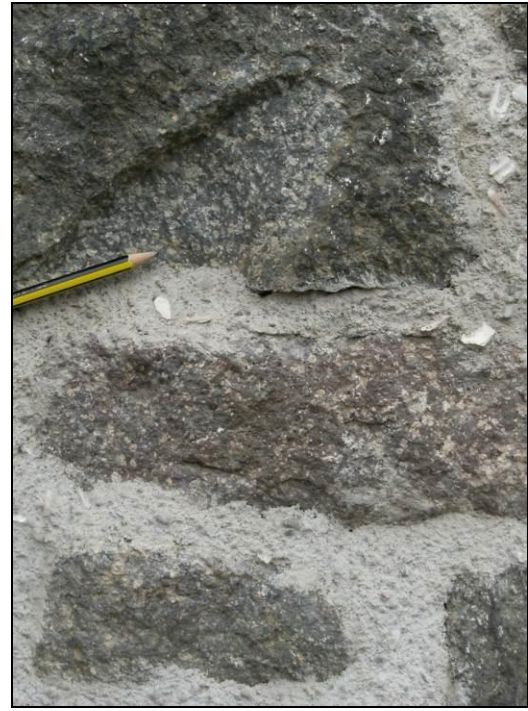
Photo ELC_12 P3: Close-up of porphyritic trachyte blocks used in the John Gray Centre. Note the large pale-coloured crystals (phenocrysts) scattered within a fine-grained dark green/purple groundmass. Typical of the material seen in Peppercraigs Quarry. © BGS, NERC.
