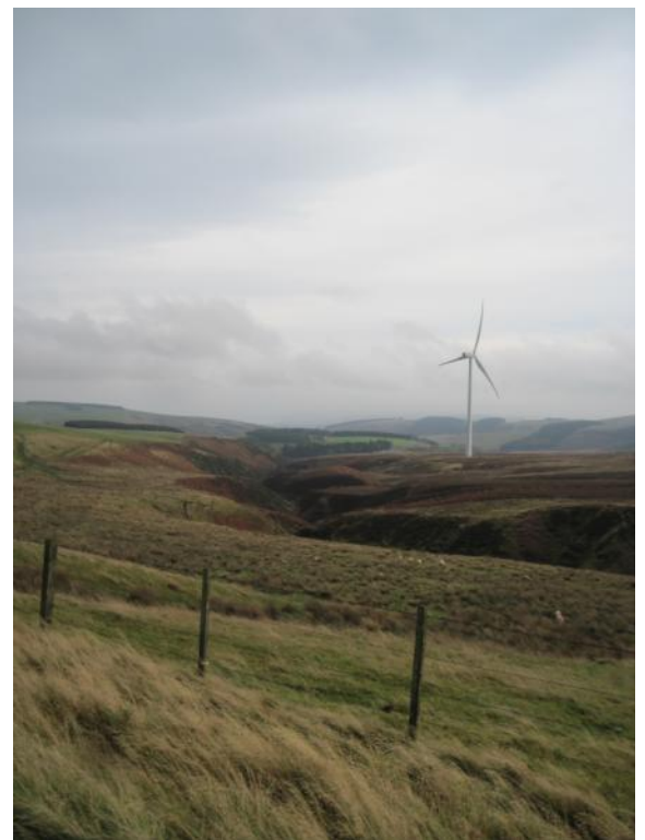
Fine open views out to the North Sea from the edges of the area. The sensitive siting of the turbines in these views creates a contrast of colour to the natural vegetation that adds to the setting and picturesqueness of the views.
