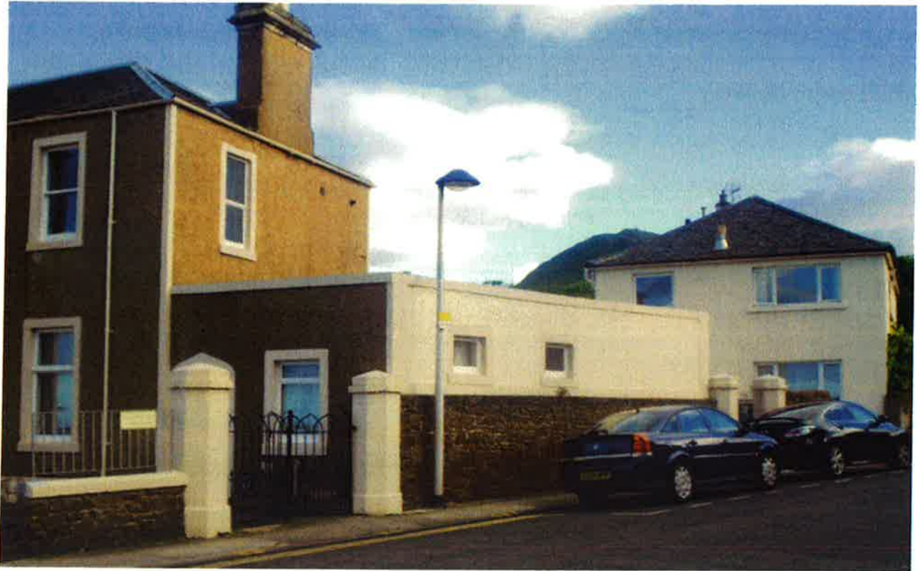
View from Quadrant / Melbourne Road / Marine Parade junction looking South East: only one window (top left) in this view is of the sash and case style
