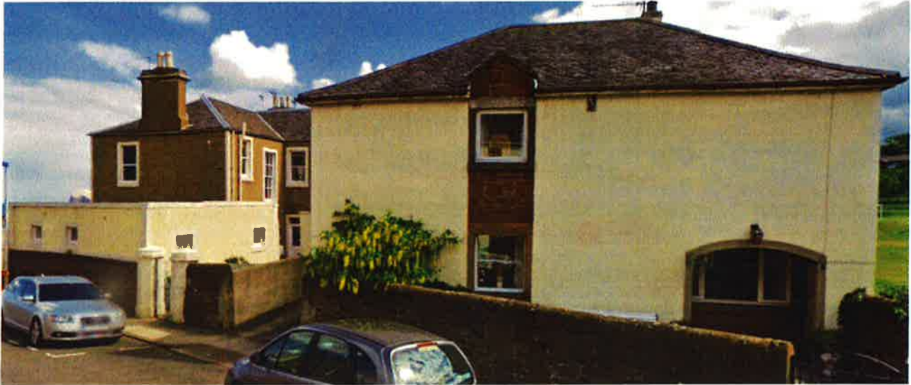
View from Quadrant looking North East showing windows of 11 Quadrant and rear of 1 Marine Parade
