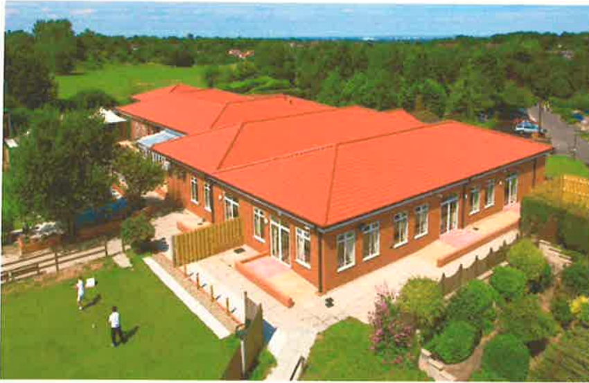
This is a profiled metal sheet roof on a golf club in England
