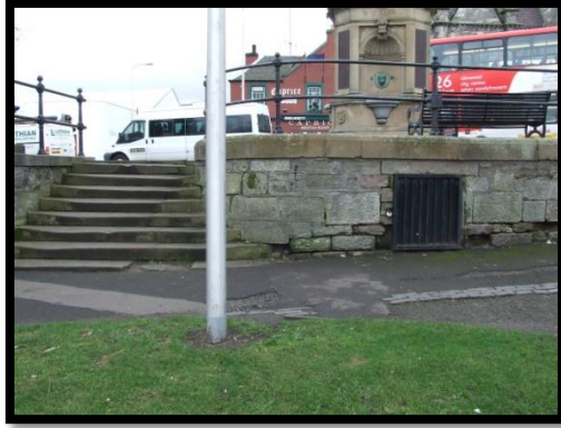
Steps and wall at War Memorial
