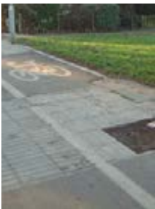
Tactile surfaces increase complexity and maintenance liability
