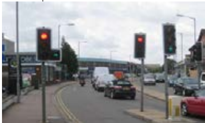
Bus pre-signal with permanent green for cyclists (requires authorisation), Cambridge
