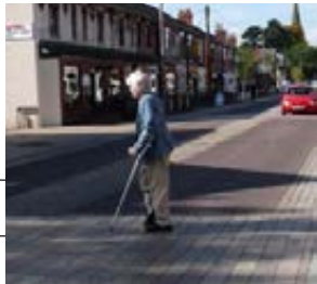
Central margin strip and informal crossing point to assist pedestrians, Poynton
