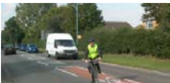
Right turn pocket for cyclists, 1.5m min width (refuge optional where width allows), Shrewsbury
