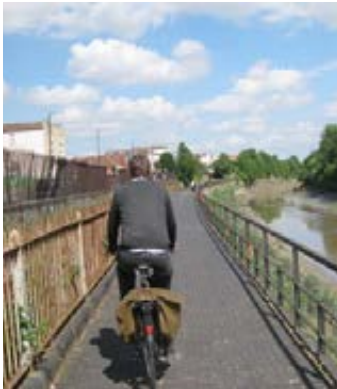
Sub-standard parapets on cycle route, Bristol
