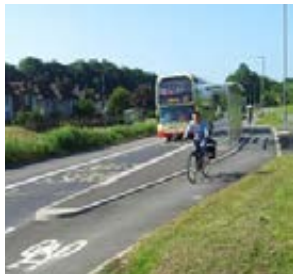
Cycle bypass at bus stop, Brighton
