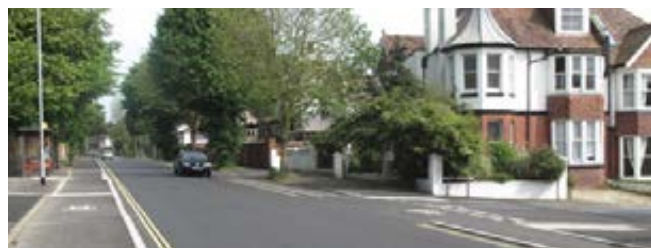
One way hybrid cycle tracks on both sides of carriageway, Brighton
