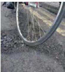
Repair damaged surface
