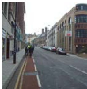
On gradients where space is limited consider provision of a wider cycle lane in the uphill direction only, Bristol
