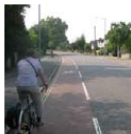
Narrowing of traffic lanes/ removal of centre line, Cambridge
