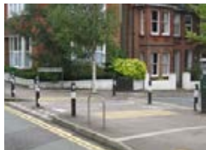
Road closure "except cycles", Brighton
