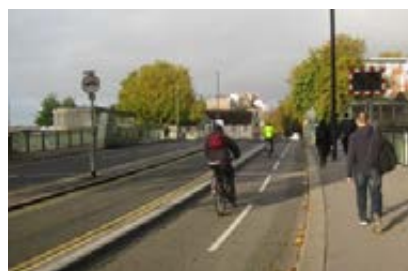
Removal of traffic lane to provide cycle track, Bristol
