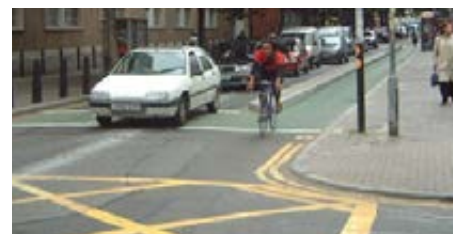
Advanced stop line with feeder lane, London
