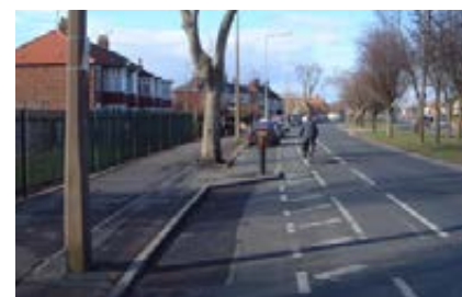
Removal of traffic lanes to provide cycle lanes, Hull
