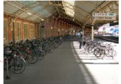
Cycle parking on platform, Bristol
