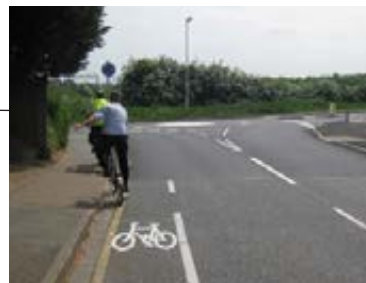
Cycle lane stops 20-30m before roundabout so cyclists mix with traffic on approach, Leighton Linlade
