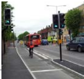
Cycle bypass at traffic signals, Brighton
