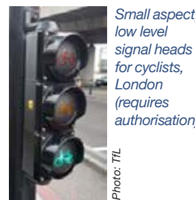
Green cycle pre-signal gives 5 seconds head start for cyclists, Examples in Brighton, York and Cambridge (requires authorisation)
