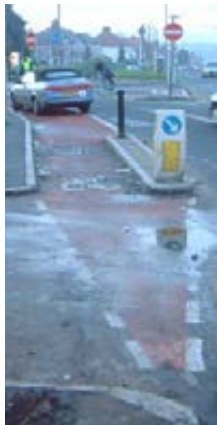
Design complexity causes maintenance liability
