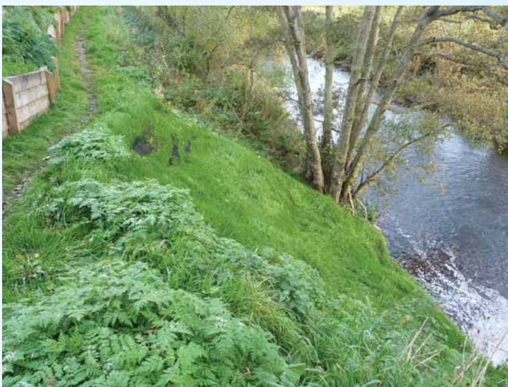
'Soft' engineering bank repair
