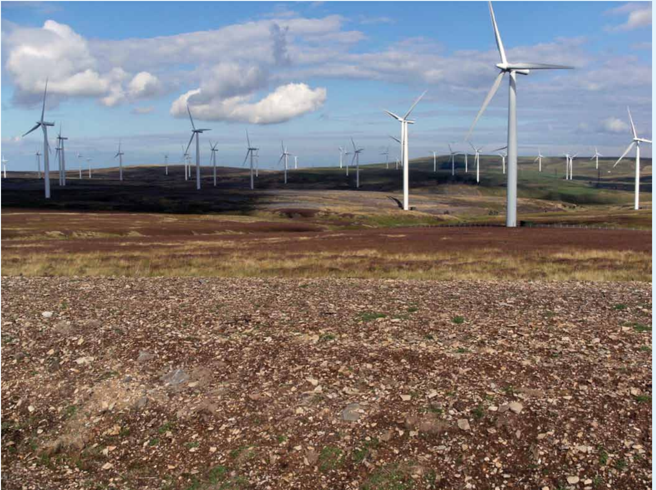
Crystal Rig wind farm
