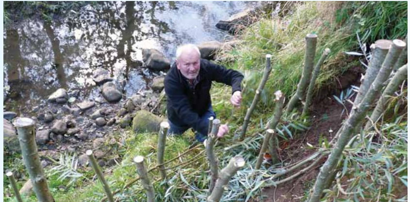
Building willow sets to prevent bank erosion
