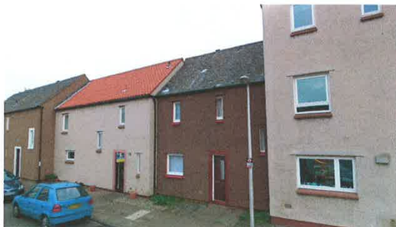
Above – PVCu windows on Lamer Street, adjacent to 'The Vennel'
