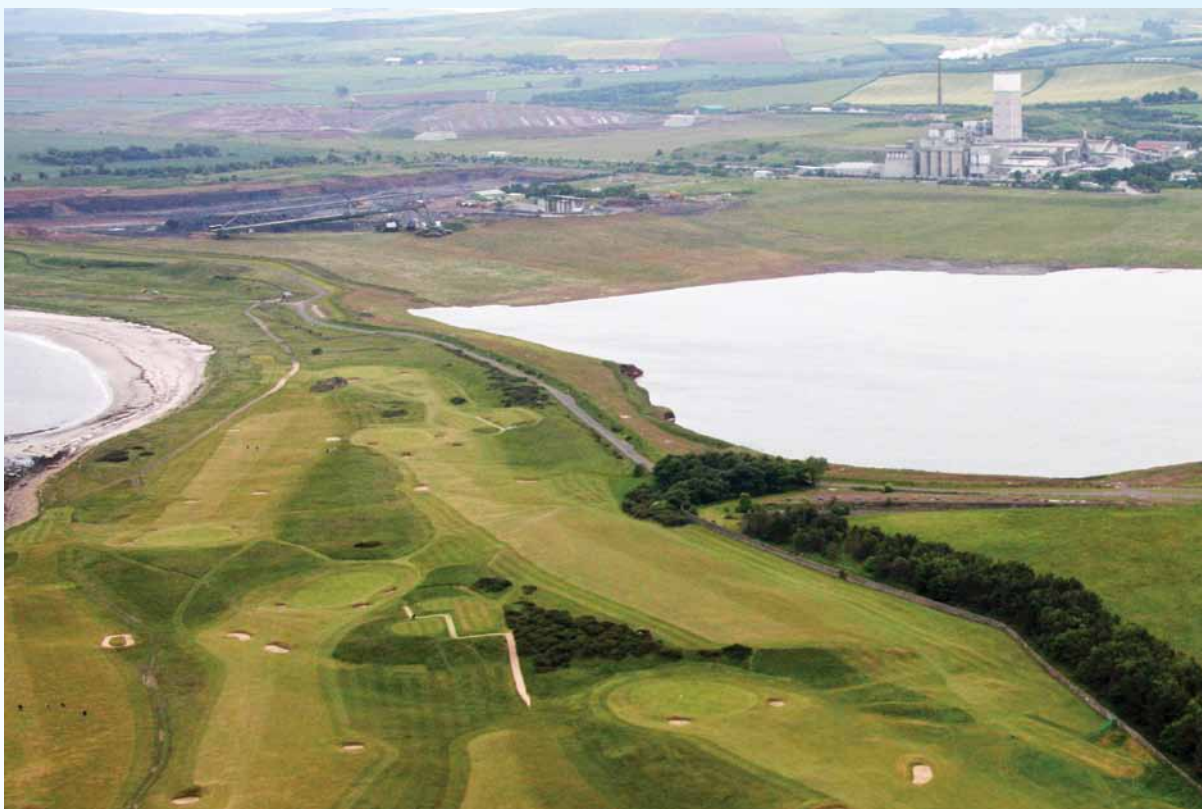
North West Quarry development
