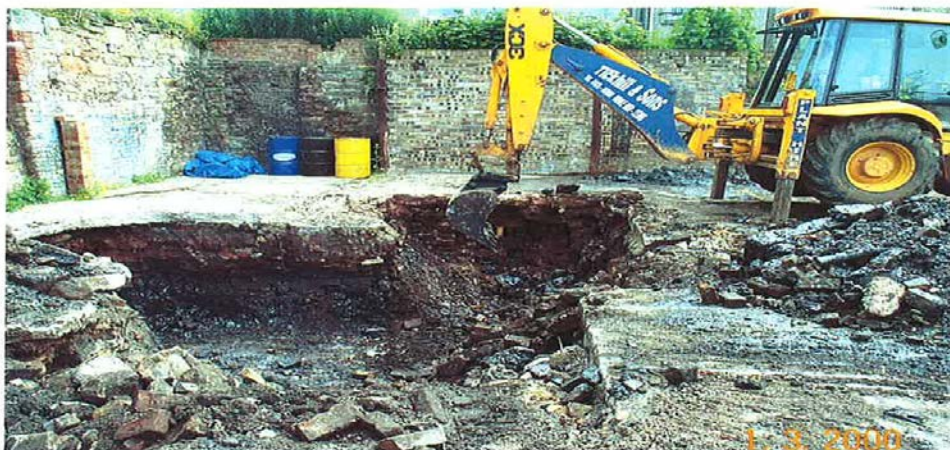
Site during Remedial Works
