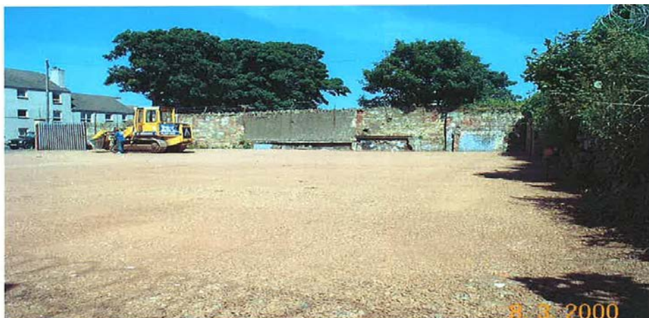
Finished, Remediated site
