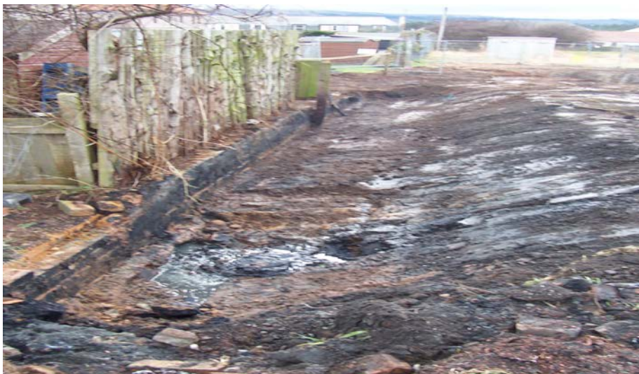
Excavations during Remedial Works
