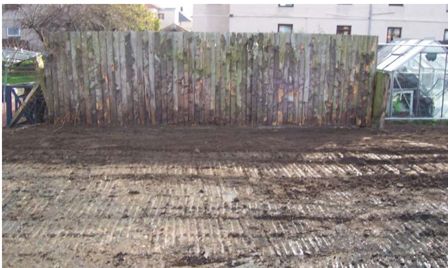
Part of the completed Site
