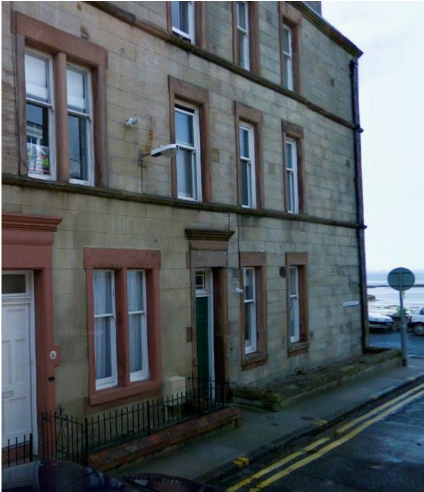
Above – 27 Balfour Street (neighbouring property, non-timber windows)
