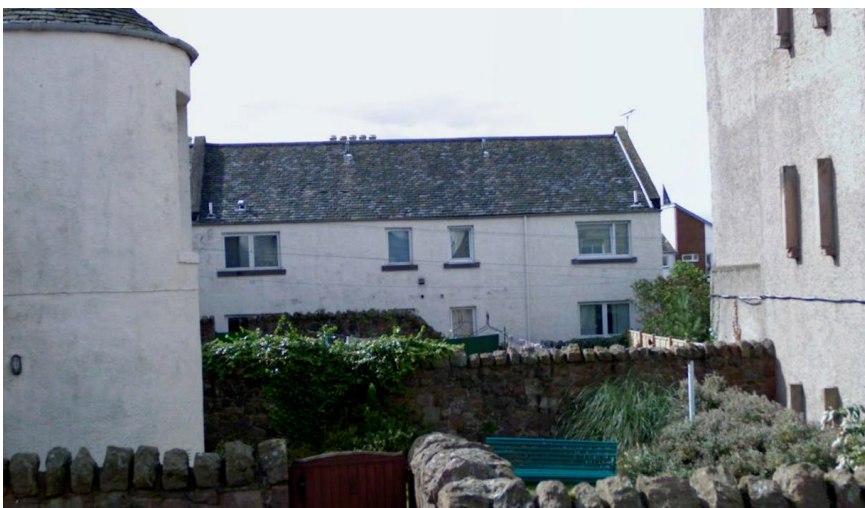
Above - PVCu windows at Brodie Court, clearly visible from Balfour Street
