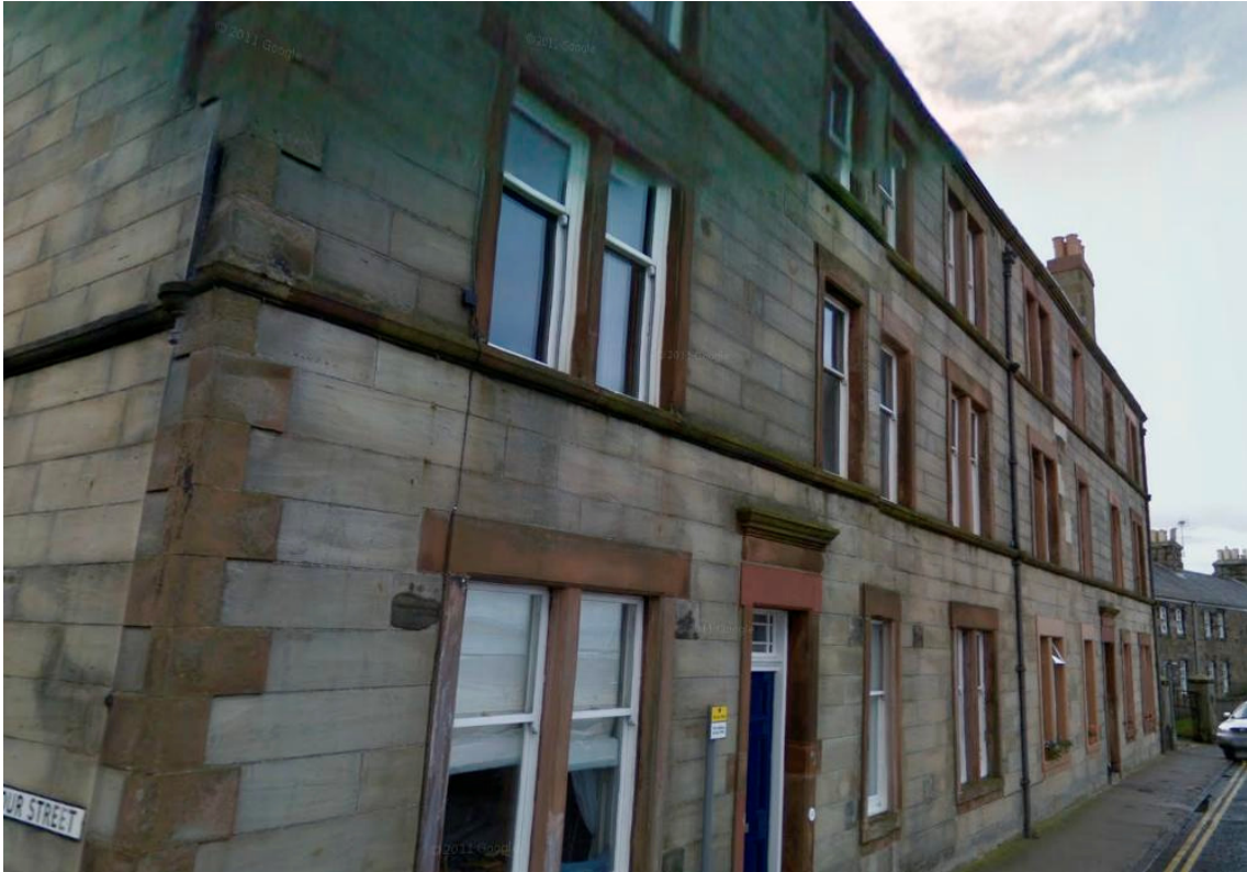
Above – Non-timber windows in a property on Melbourne Road, off Balfour Street
