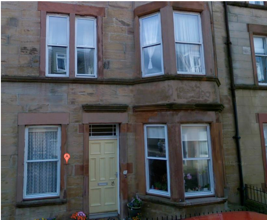
Above – 23 Balfour Street (non-timber windows)
