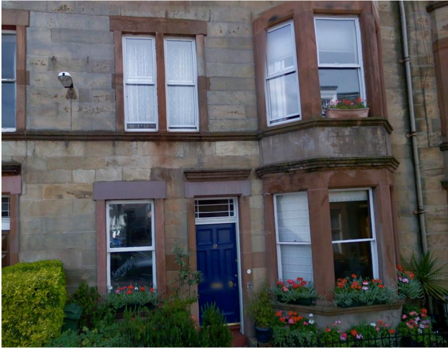
Above – 17 Balfour Street (non-timber windows)
