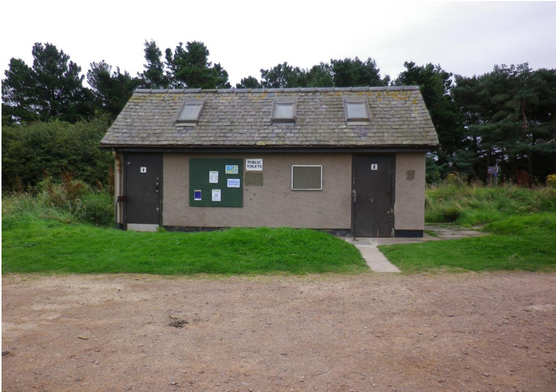
Longniddry No 2 Toilets
