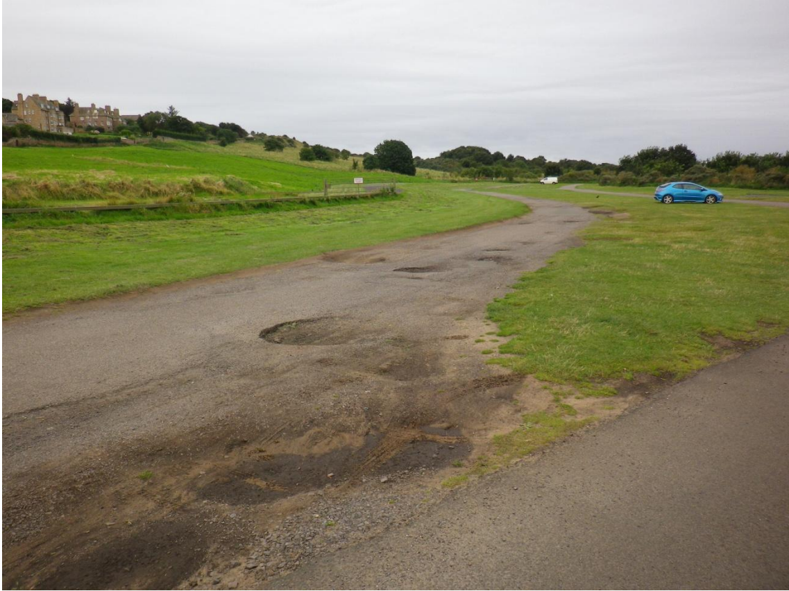
Gullane Bents Car Park Internal Road
