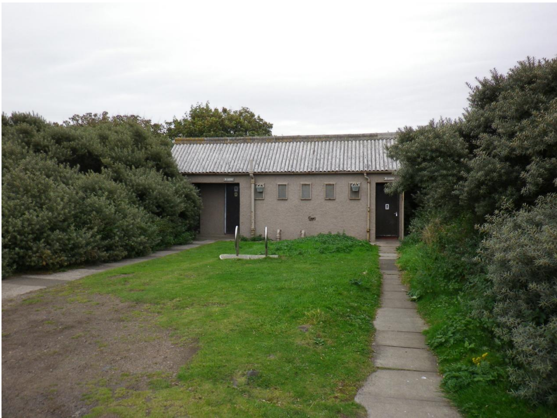
Longniddry No 3 Toilets
