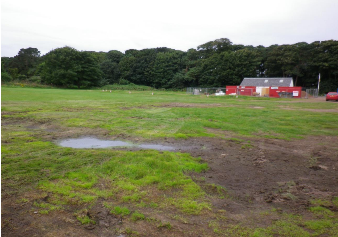
Yellowcraig Car Park Surface
