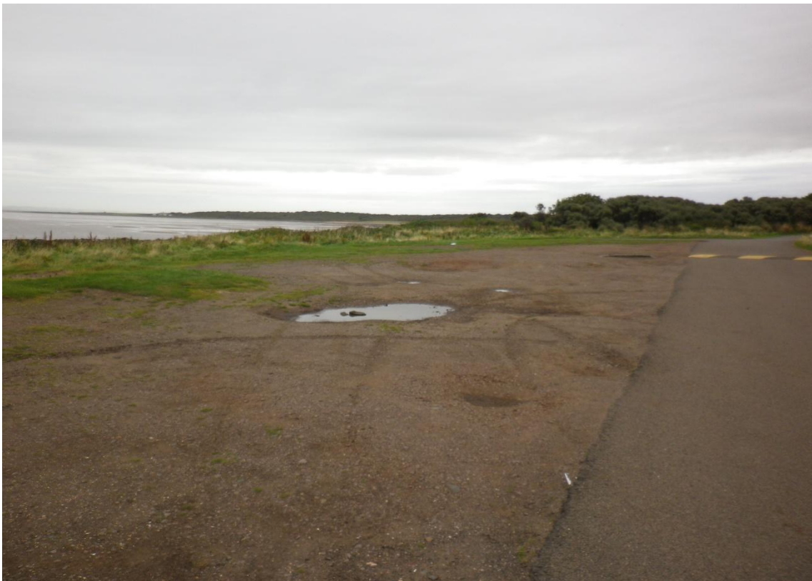
Longniddry No 3 Parking Surface
