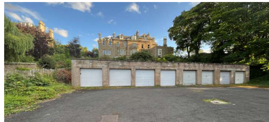
GARAGE COURTS SITE 3 - CROMWELL ROAD
