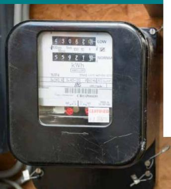
The RTS uses a radio signal to tell some older electricity meters when to switch between peak and off–peak rates. It was introduced in the 1980s and is now reaching the end of it's operational life, in June 2025.
