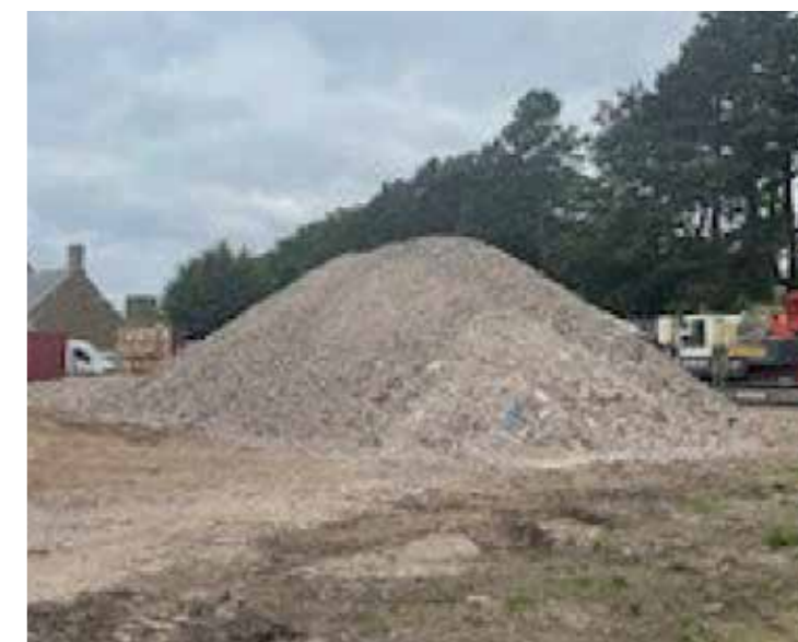
Demolition rubble retained for re-use
