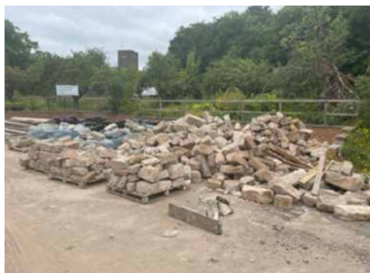
Stockpiling on site of demolition rubble for re-use
