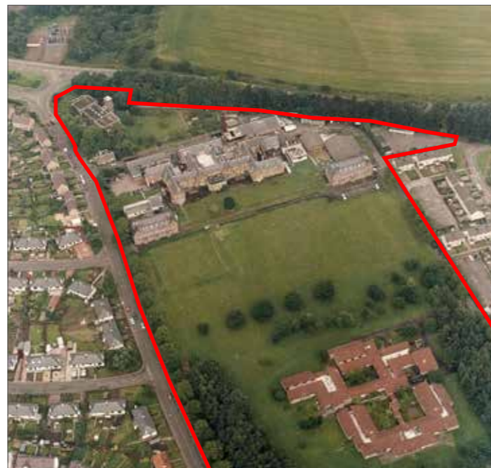
Construction of Hopetoun Unit and ancillary hospital buildings
