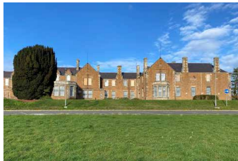
Reflect and enhance existing formal areas to provide social spaces around the main building
