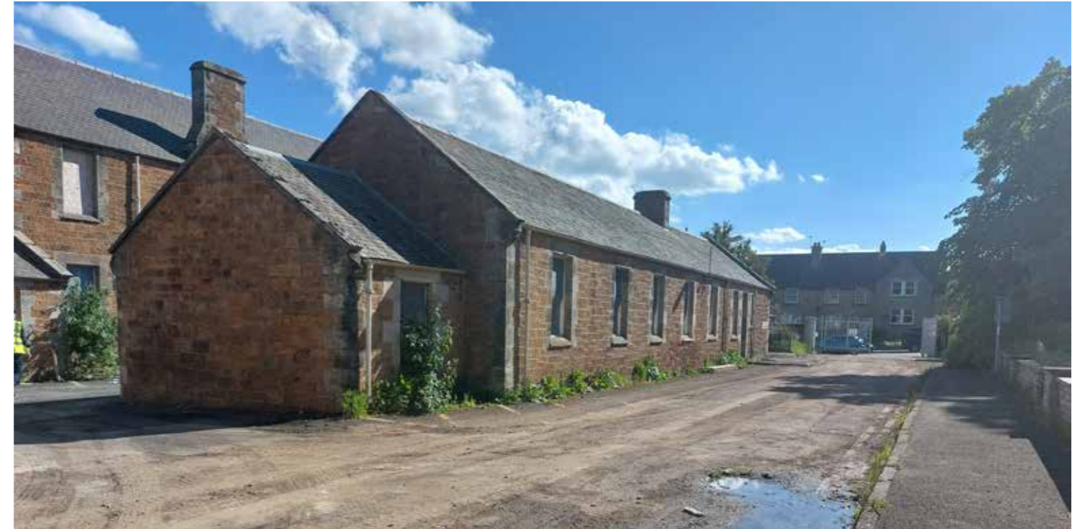
Ancillary Building, former Herdmanflat Hospital, Category C Listed
