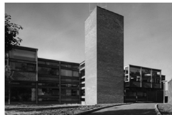
The Garleton building shortly after completion in 1965
