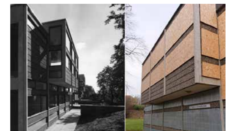
Garleton shortly after completion in 1965, and the same elevation in 2023
