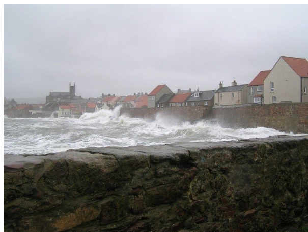
Picture 5.1: Flood damage to properties on Lammer Street, Dunbar, courtesy of Alex
