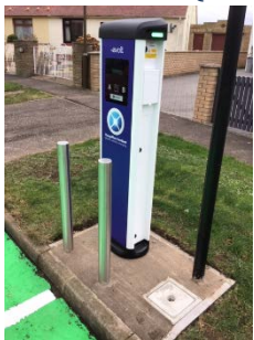
Figure 4: Example Destination (Fast) chargepoint
